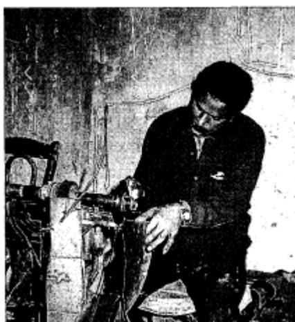
**Figure 7.4 Cutting Inner Tubes into Elastic Cords, Cairo, Egypt**
